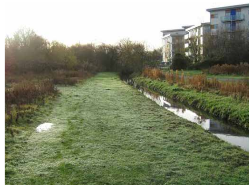
This image shows adequate access to effectively maintain SuDS features.
