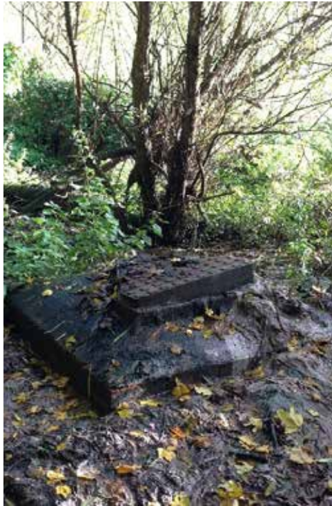
This image of a sewer overflow is the result of overstressed water infrastructure. One advantage of SuDS is their ability to remove surface water runoff from the sewer system, improving its capacity for managing wastewater.
